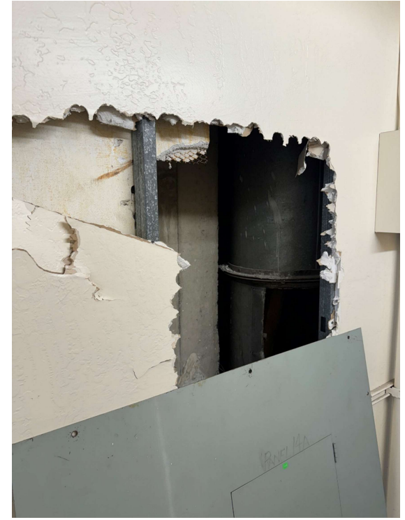
Sampling of materials in and behind walls for hazardous materials
