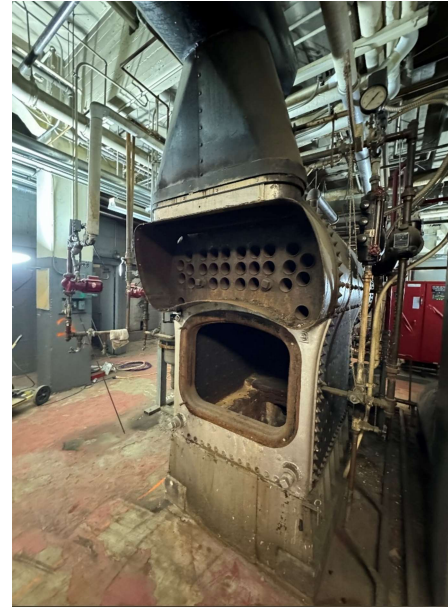
Boiler doors removed
