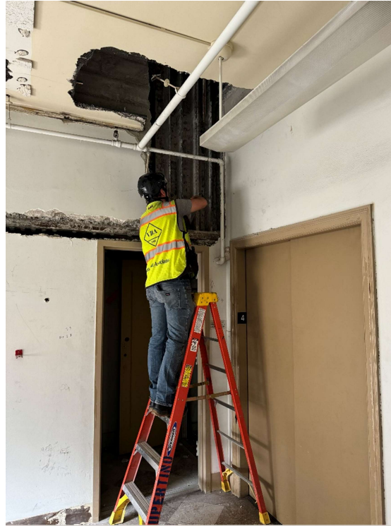
Taking samples of paint on structural steel
