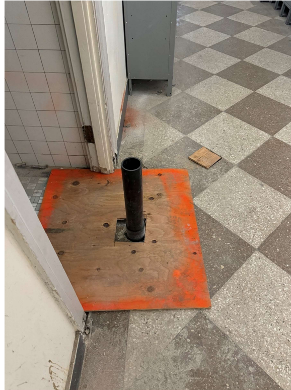
Taking additional soil samples at the basement level to confirm foundation improvement cost estimates
