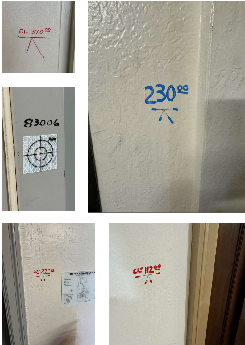
Interior floor elevations surveyed at each level
