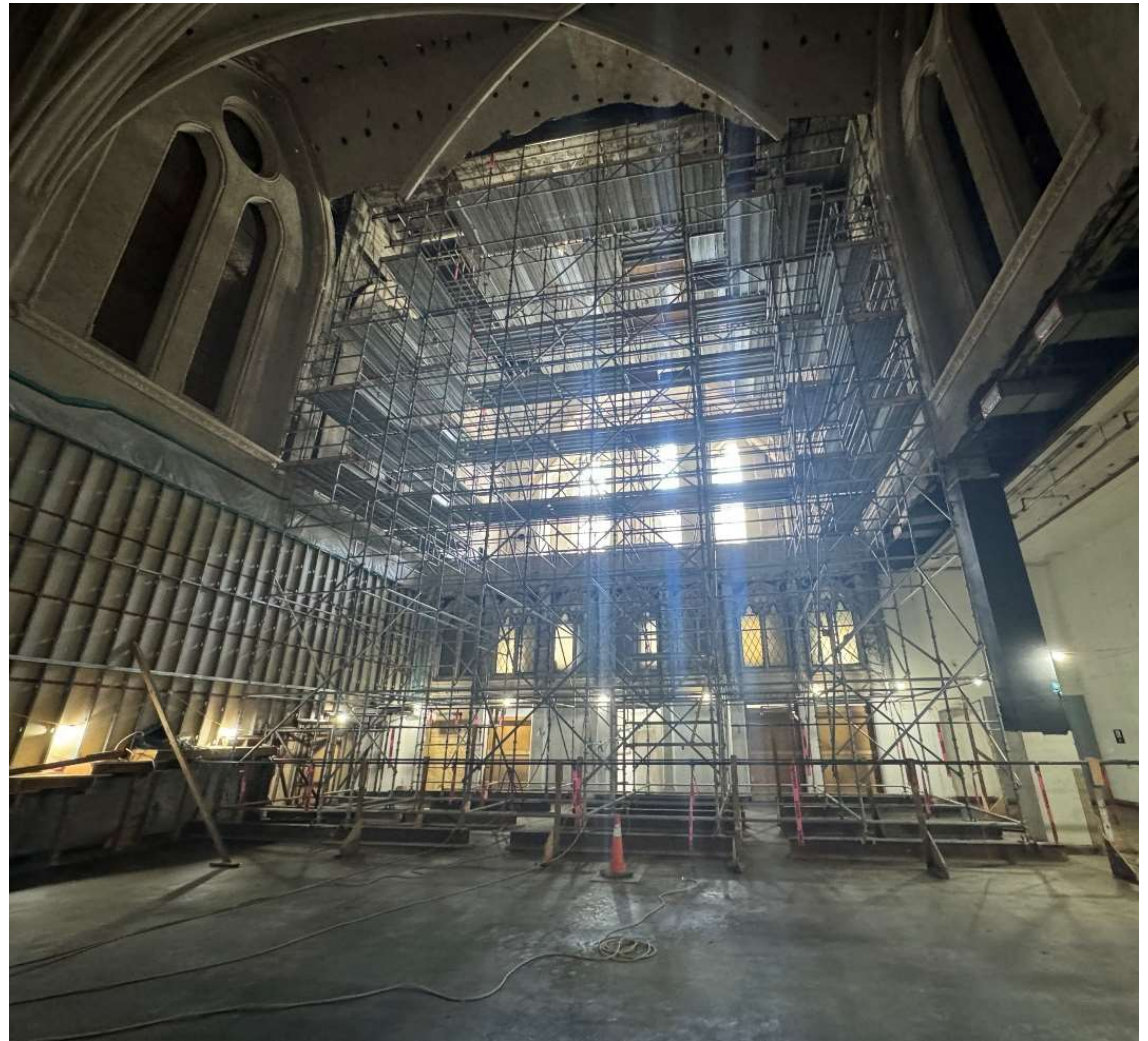
After demo and abatement of risers and stage
