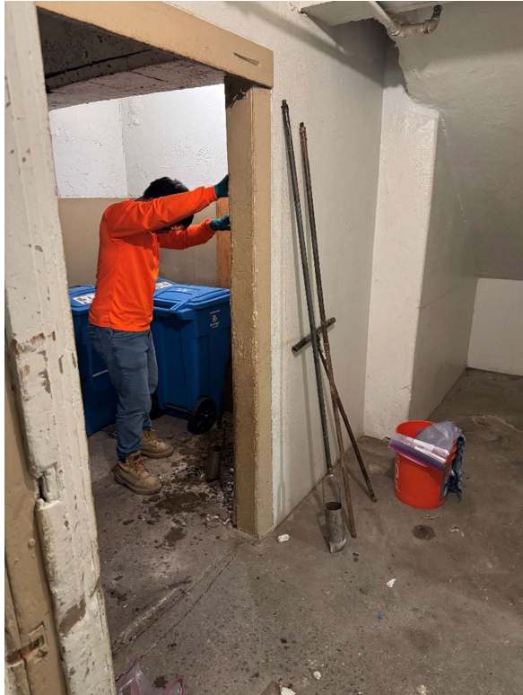
Taking additional soil samples at the basement level to confirm foundation improvement cost estimates
