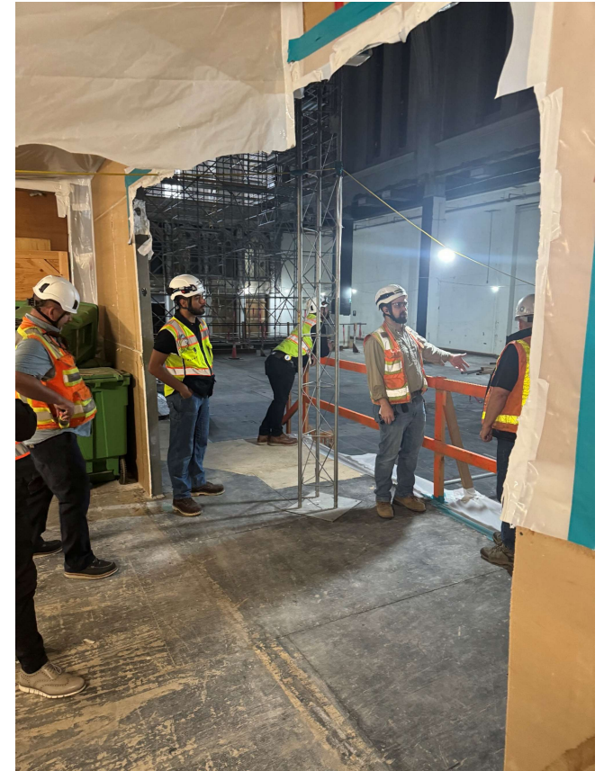
Walking with subcontractors to validate approach to structural demolition
